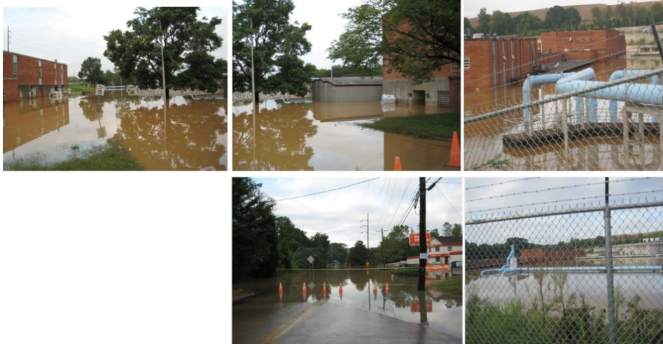
Figure 2. 2009 Flooding at RM Clayton Water Reclamation Center
